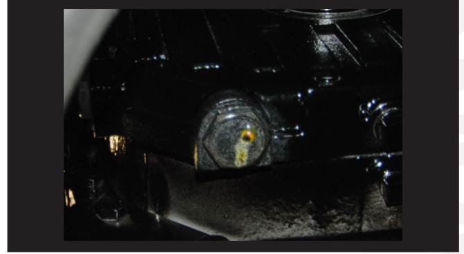
Blower Drain Valve (two drain valves located on the bottom)
